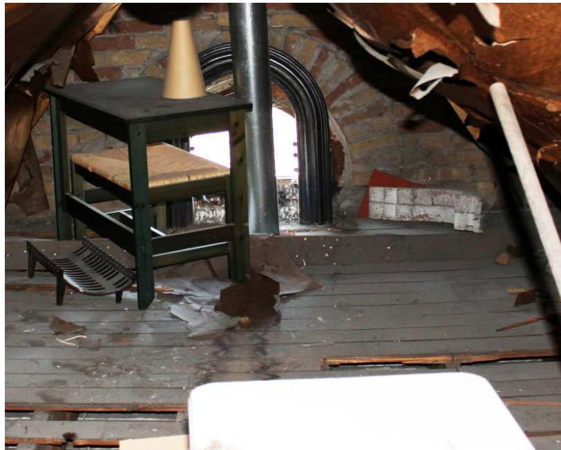
Side attic window from inside looking out.
