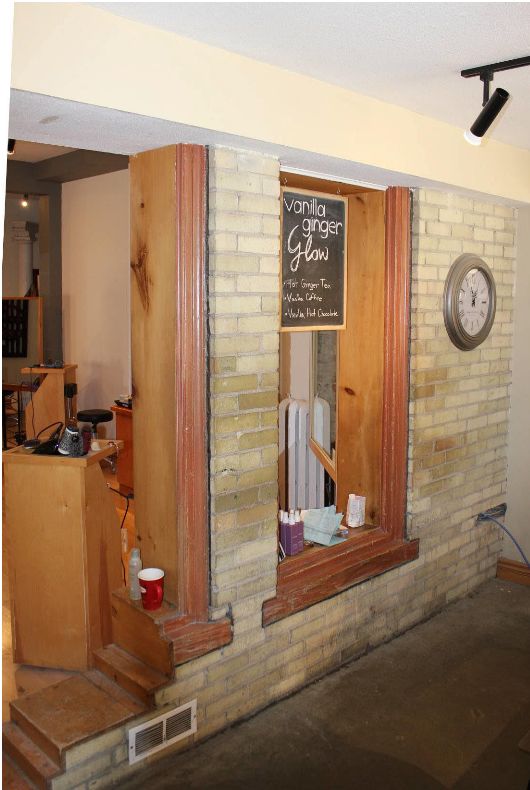
Front porch windows, one of which has been modified as a door into the main part of the building. (c).
